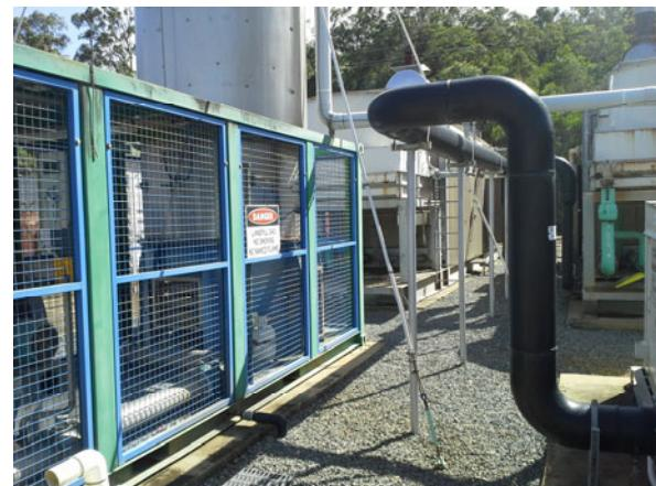
Specific attention was given to the potential methane hazard where a failure of the extraction system and leaky equipment could create a build-up of methane inside the module. This was addressed with the design and implementation of a SIL2 rated functional safety system.
